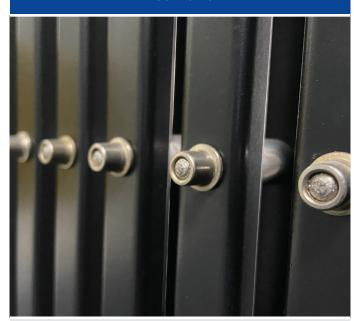
• Huckbolt fixings. Additional strength against tampering, attack and stresses caused through crowd-loading.
